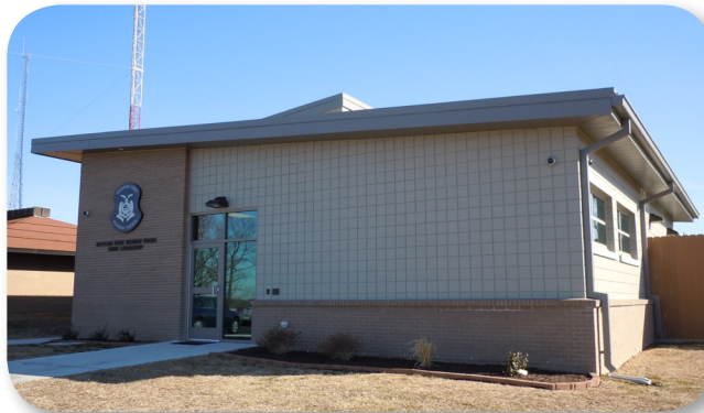
Pictured is the new laboratory at the Troop D Service Center in Carthage, MO.
