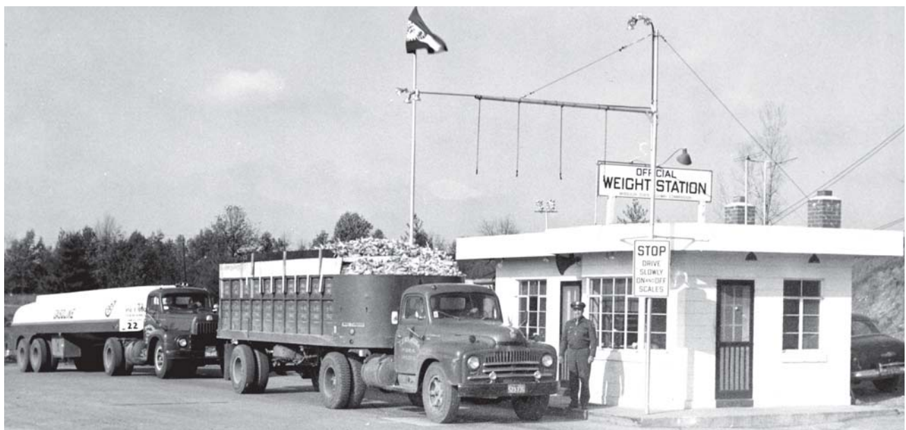
Weight Inspector Herb Lee at work in Kingdom City on November 22, 1954.
