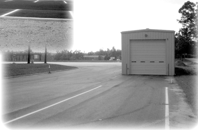
Commercial drivers began using this drive-through garage during their CDL exam (Troop I).
