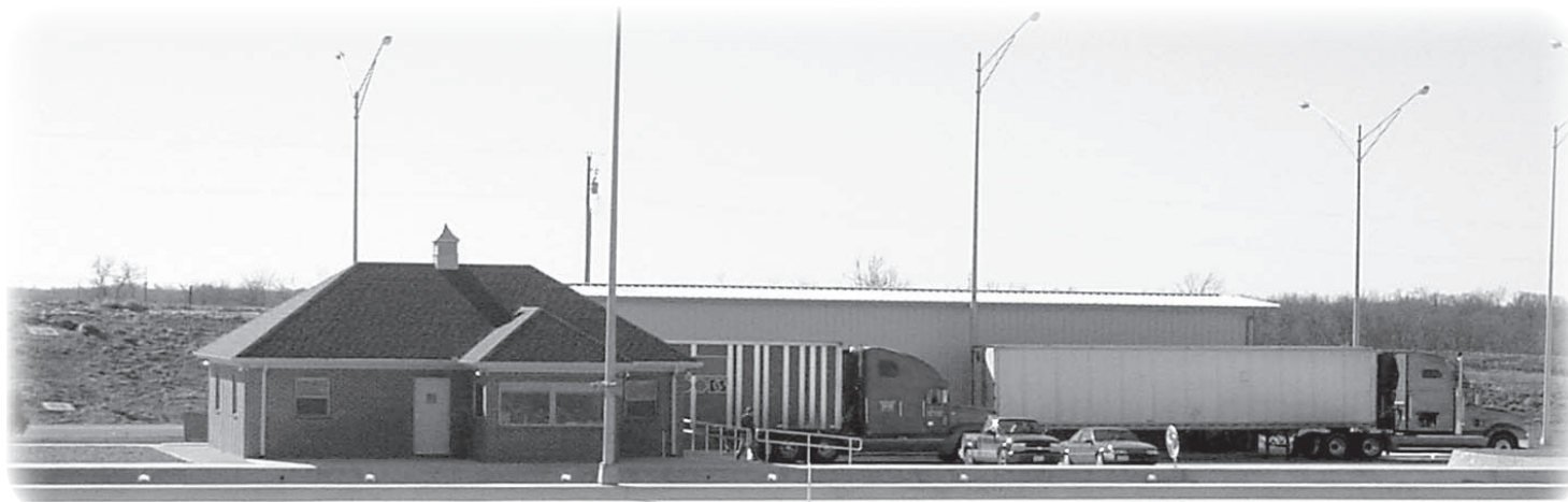
Pictured is the new A-3 scale house near Mayview, MO.
